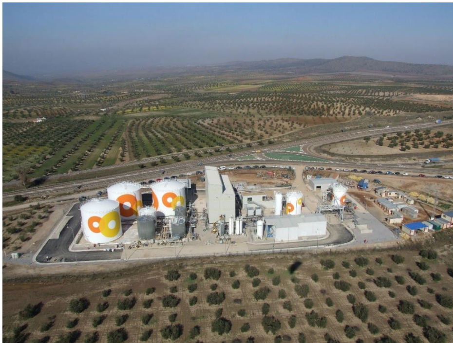
Figure 2. Aerial image of the plant.
