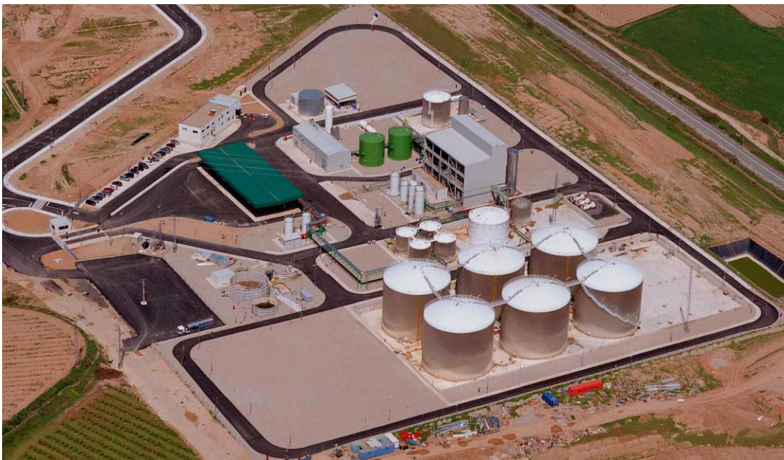
Figure 1. Aerial image of the plant.
